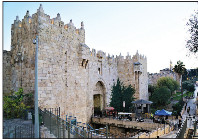
THE DAMASCUS GATE IN JERUSALEM'S NORTHERN WALL: In biblical times, this gate opened onto the road that led to Damascus, Syria. - [Photo by Chip Thompson, 2022]
